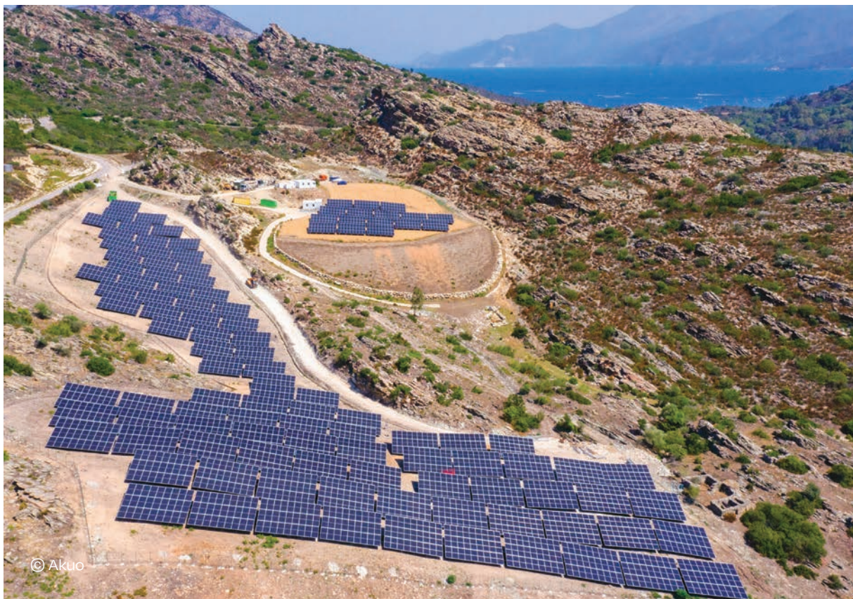
1.7 MW PV coupled with 5.2 MWh BESS, Pleve, Corsica, France
