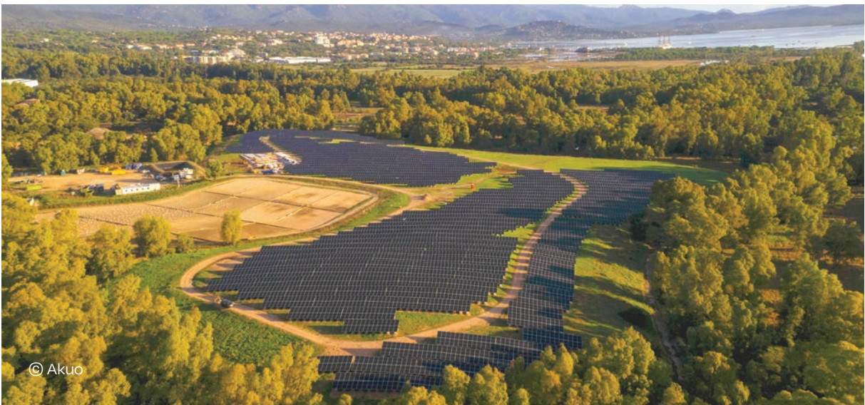
5.1 MW PV coupled with 16.1 MWh BESS, Porto-Vecchio, Corsica, France
