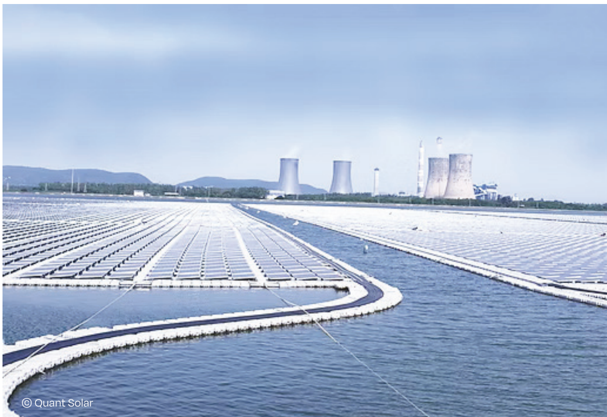
36 MW Floating Solar Project, Visakhapatnam, India
