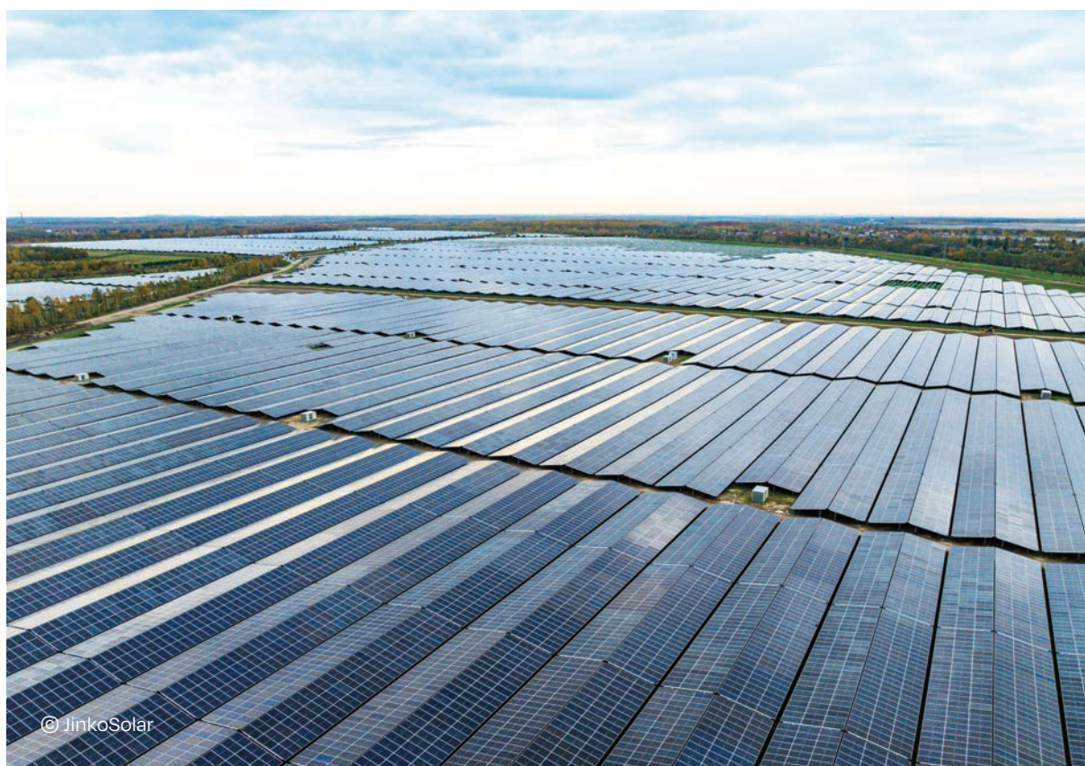
650 MW, Witzniz, Germany
