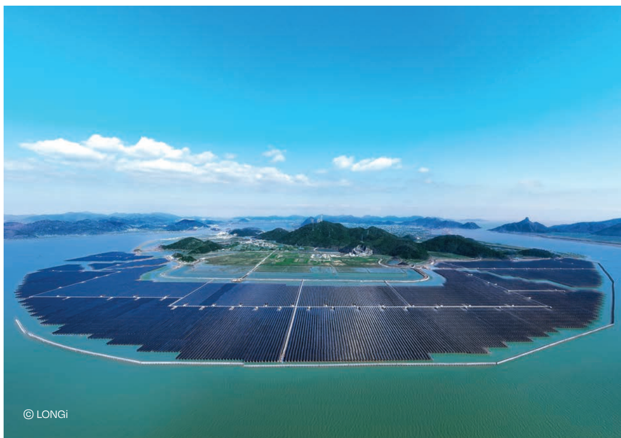
300 MW solar project, Ningbo, Zhejiang province, China
