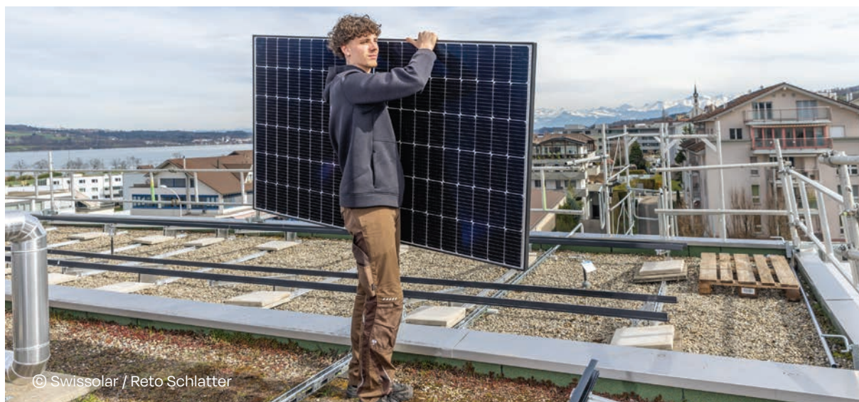
Solar apprentice working on a roof
