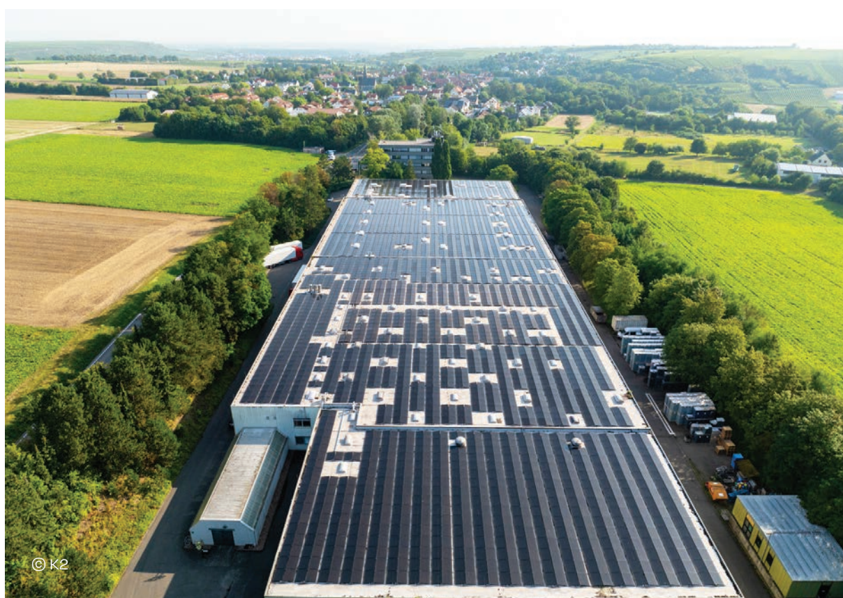
2 MW rooftop solar on wine cellar, Dexheim, Germany
