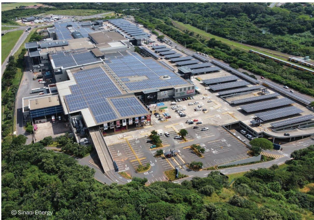
3.6 MW Galleria Mall solar rooftop and carport system, South Africa
